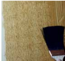
Fig. 2 Creating the wood pores with the flogger.
